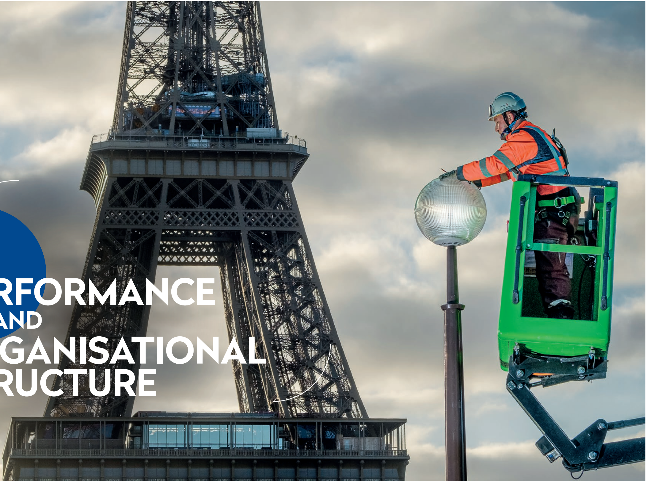
Lamp post refurbishment in Paris, France.
